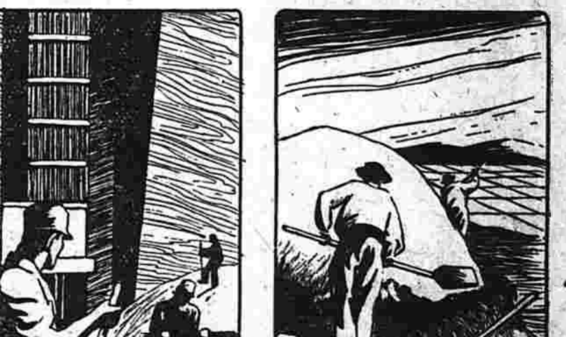
Workmen here are covering a heap of salt with clay to protect it from the rain. This is a custom in the south of Europe.
